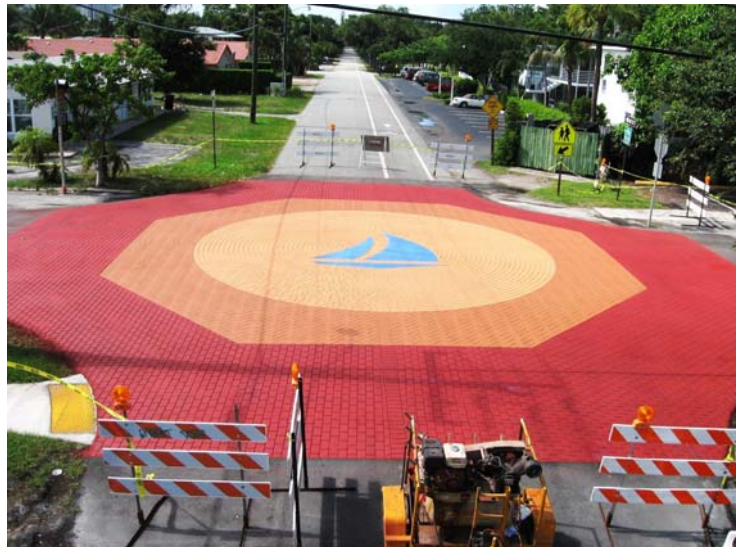
Spectacular view of 10th Ave & 15th Street intersection project.
